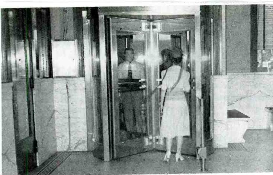
Revolving door with photoelectric control, in the American National Bank, Vincennes, Indiana
